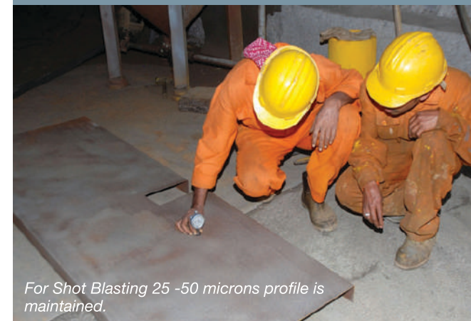
DFT (Dry film thickness) checking and Holiday test being carried out.
